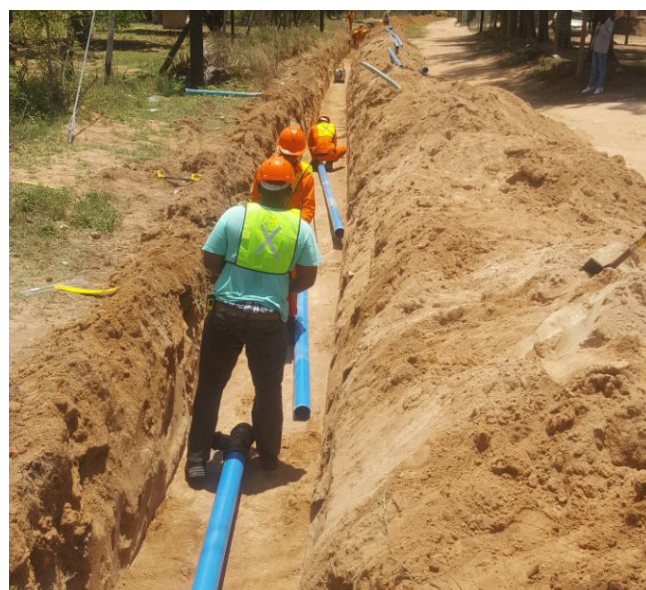
Some of the contractors working on the water reticulation project
