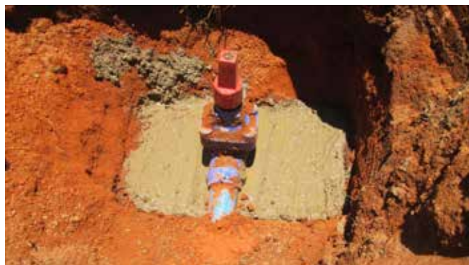
Isolation Valve Construction Maviljan A,B and C Water Reticulation Project Phase 3
