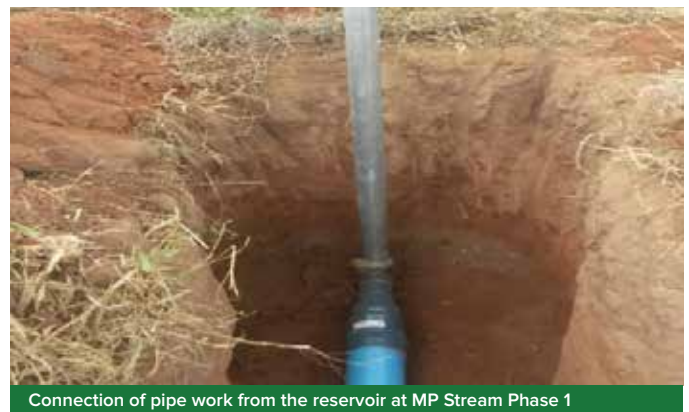
Connection of pipe work from the reservoir at MP Stream Phase 1
