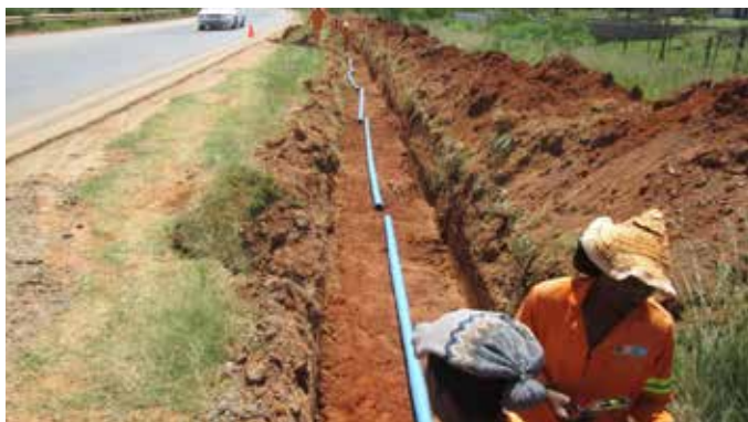
Pipe laying works Maviljan A, B, C Water Reticulation Project Phase 3
