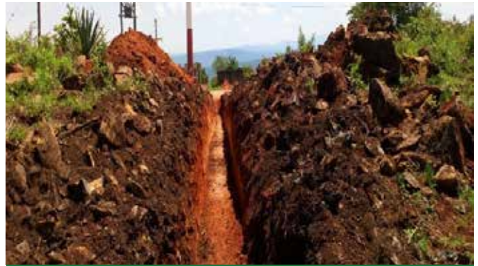
Water reticulation at Sandford
