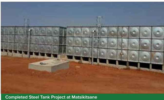
Completed Steel Tank Project at Matsikitsane
