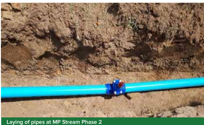
Laying of pipes at MP Stream Phase 2
