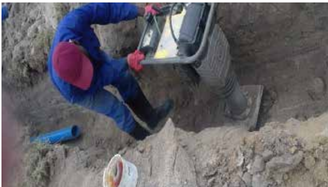
Water Project underway at MP Stream Phase 3
