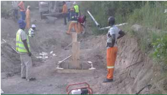
Water Project underway at Maromeng Phase 2
